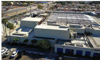
Mexicali, Mexico Back End Assembly and Test
